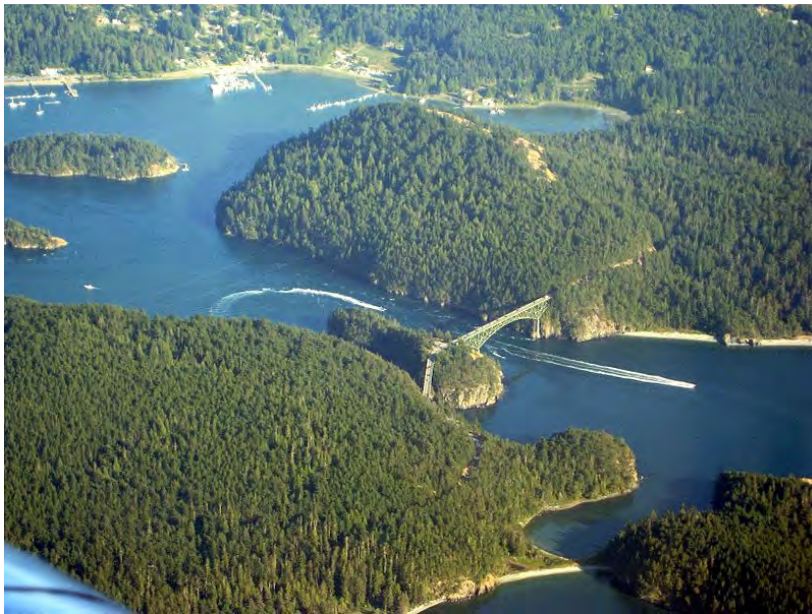
Aerial View of Deception Pass, including the Bridge and State Park [Photo: Wikipedia]
