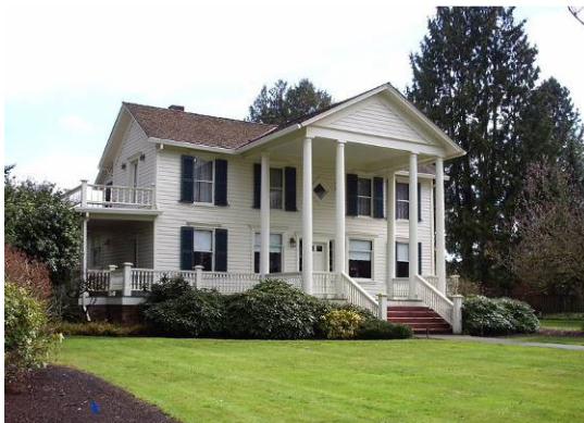
← The Joel Palmer House, built in the 1850s, is one of the Beaver State's finest restored historic homes. It's named for one of Dayton's pioneer settlers.
