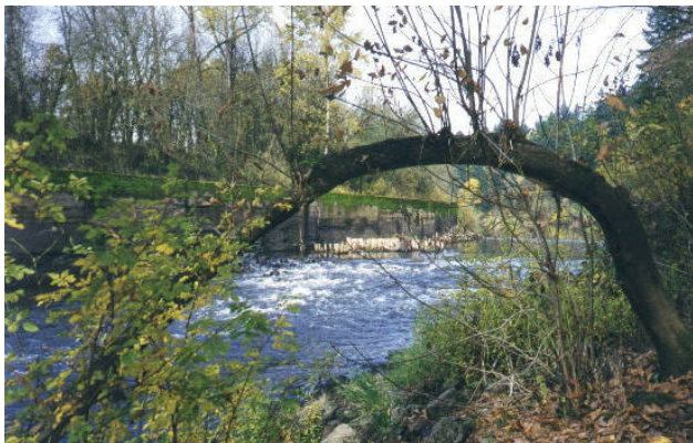
Concrete lock walls at Lafayette Locks County Park [Photo: Yamhill County Parks]
